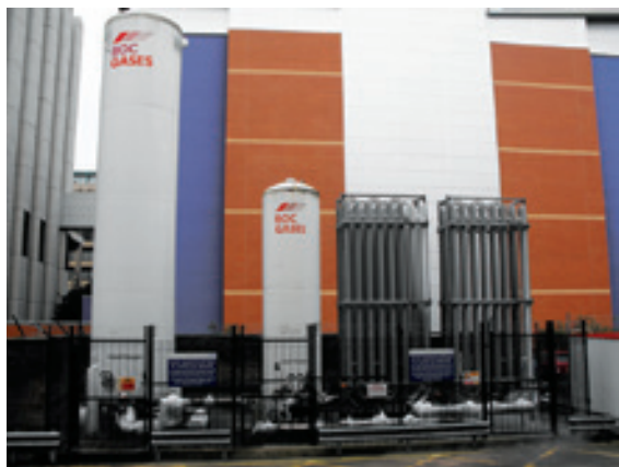
FIGURE 1-1 Liquid oxygen vessel used for bulk storage for an acute care facility. This illustration shows the bulk oxygen vessel at a distance from the facility surrounded by a protective fence, lighting, and signage.
