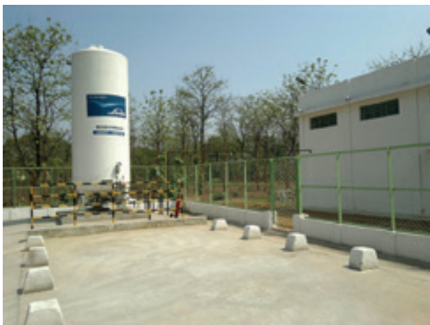
FIGURE 1-3 The NFPA Health Care Handbook provides guidelines for minimum distances for locating structures around bulk oxygen supplies.
