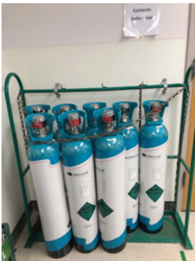
FIGURE 1-17 Racks that are tethered to the wall are used to secure larger high-pressure cylinders (e.g., H cylinders). Chains are used to secure each cylinder within a holder.
