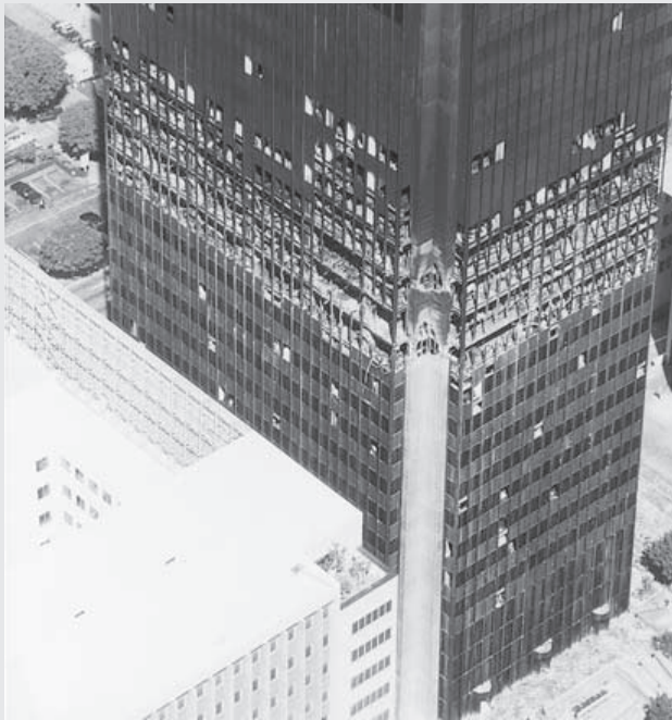
Figure 12-16 First Interstate Bank Building, Los Angeles, California.
