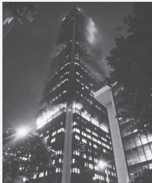
Figure CS12-1 The fire at the First Interstate Bank Building.
