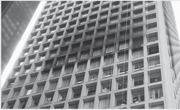
Figure 12-19 East side of 12th floor, Cook County Administration Building.
