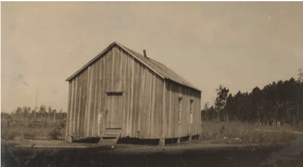
Figure 2.13 An old one-room schoolhouse.
